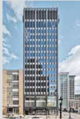
Jiakai City Building
